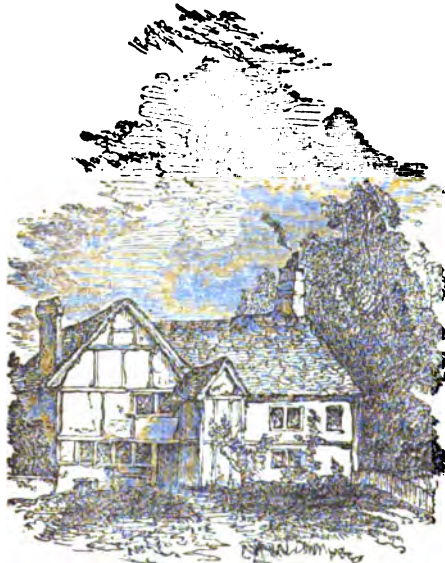
Milton's Cottage at Chalfont.
